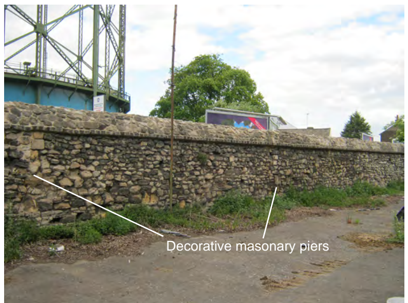
Photo 2: Possible original wall below decorative masonry pier (to left of shot)
