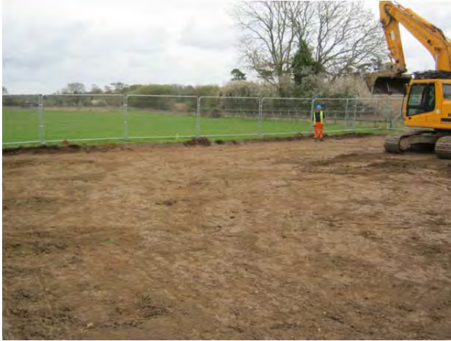
Topsoil strip of Water Treatment Works
