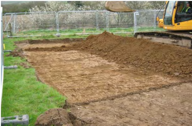
Strip of Water Treatment Works to natural horizon
