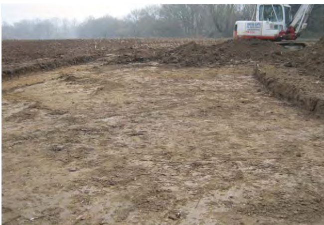
Temporary Compound topsoil strip
