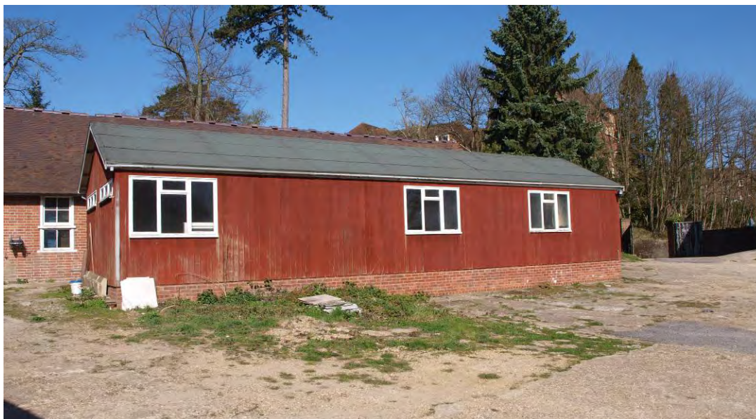
Plate 2. Building 2 from east
