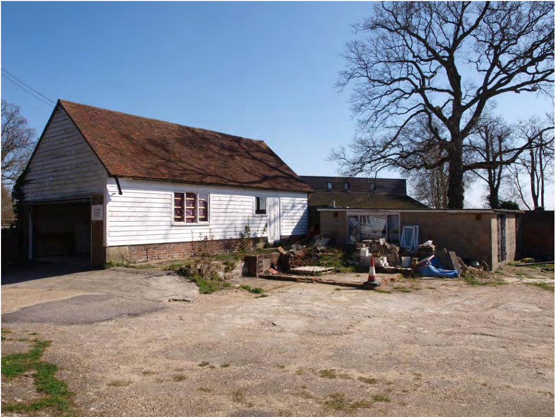
Plate 4. Building 4 and Building 5 from south-west
