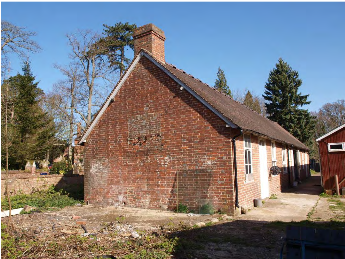
Plate 1. Building 1 from south
