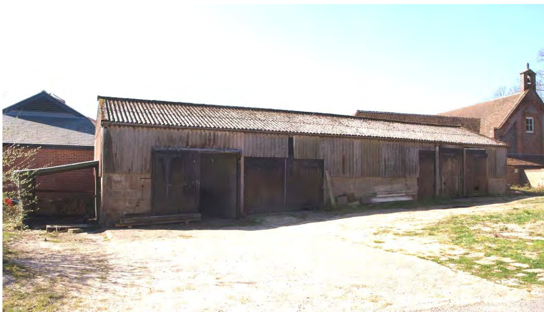
Plate 3. Building 3 from north
