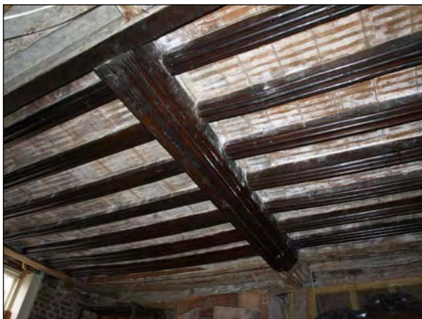
General ceiling view
