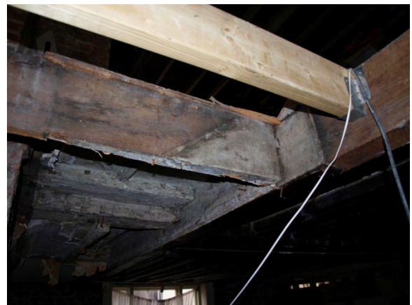
Plate 2: Main range - detail of the moulded joists in the central room ceiling shows straight cut stops at former jetty plate location
