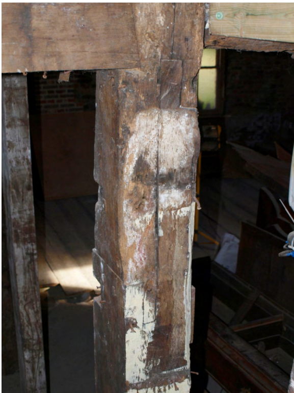
Plate 3: Main range – detail of scarfed post in Phase 2 partition wall
