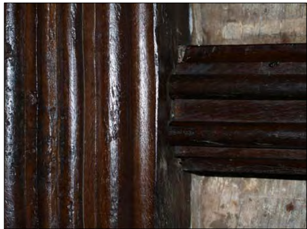
Detail of girder and joist
