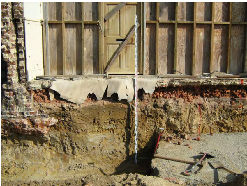
Fig. 5: North facing view of make-up under existing building
