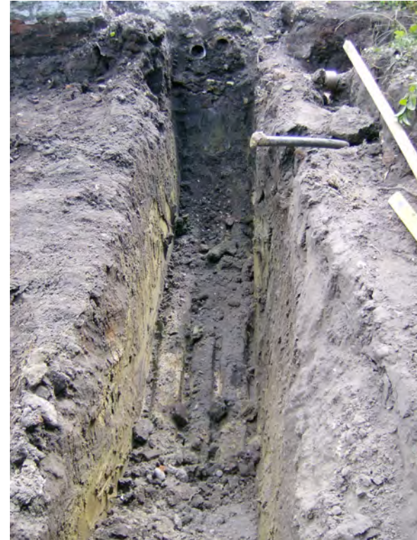
Fig. 6: Footing trench
