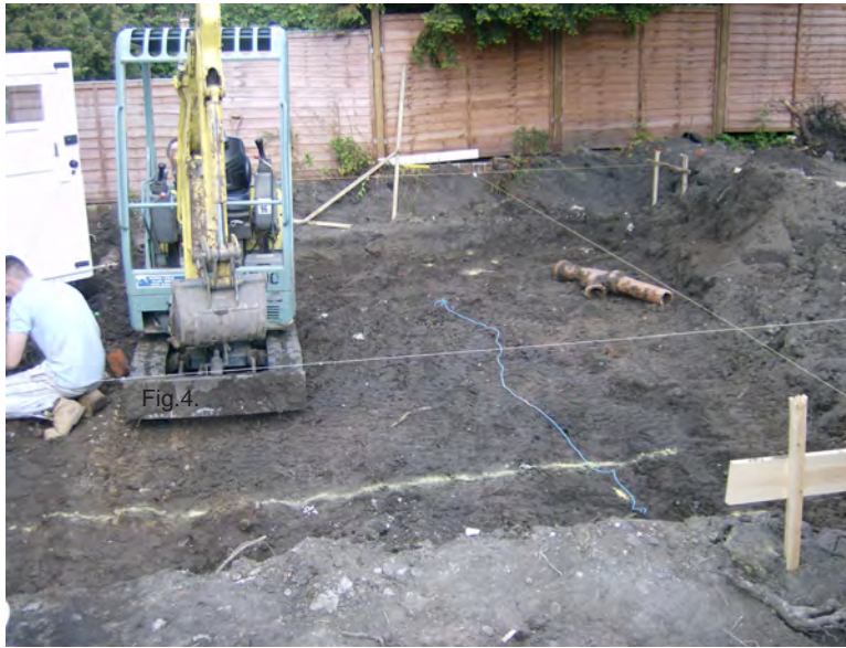
Fig. 4: Reduction of ground level in area of new build
