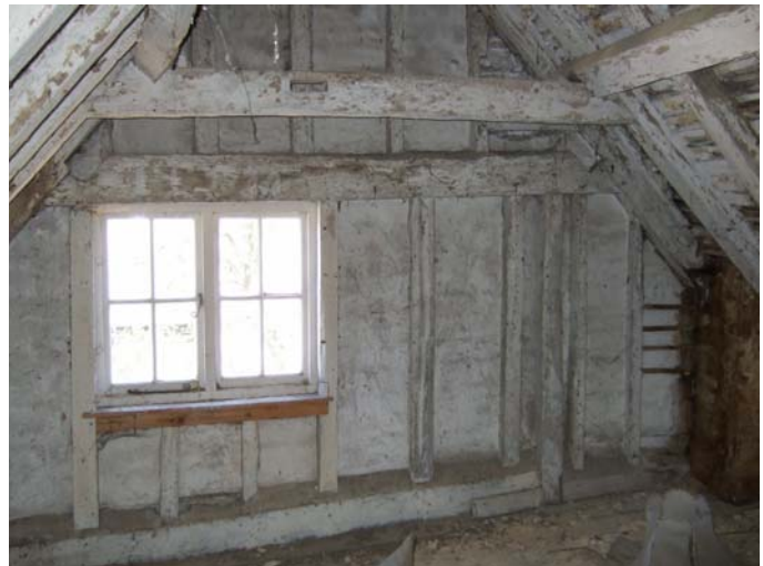
Plate 1 Period-A truss F-F showing later intermediate truss in foreground.
