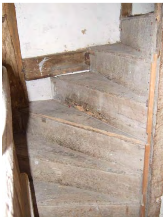
Plate 3 Staircase leading to attic.
