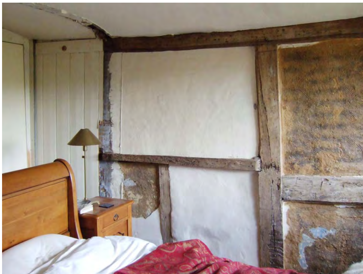
Plate 1 Blocked window in front wall of hall chamber, with remains of adjacent comb-decorated daub
