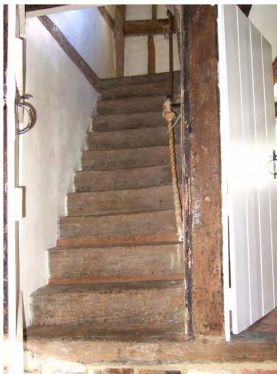
Plate 2 Triangular-tread staircase leading to first floor.
