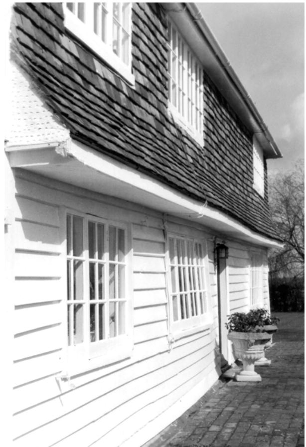
Plate 1 Methersham, Beckley, showing pentice roof.
