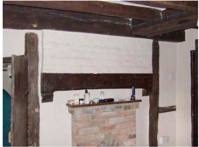
Plate 4 Kitchen chamber fireplace showing lintel supported by projecting timber corbels.
