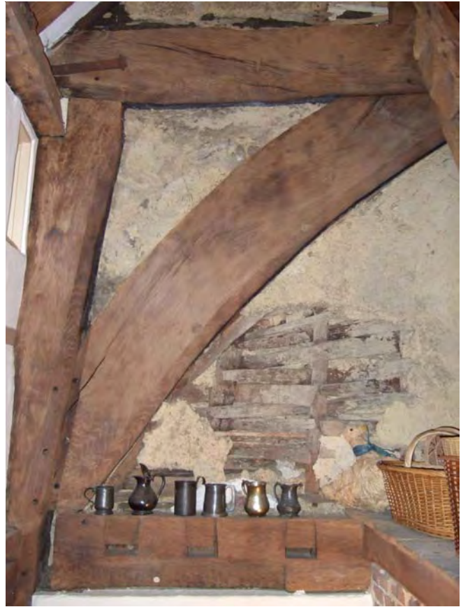
Plate 2 Surviving eastern brace of hall truss, viewed from north.
