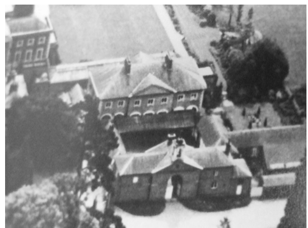
Plate 18 Courtyard complex from the west in the second quarter of the 20th century
