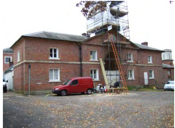
Plate 16 Main elevation of Briar and Dawn Cottages in 2007 showing additional windows
