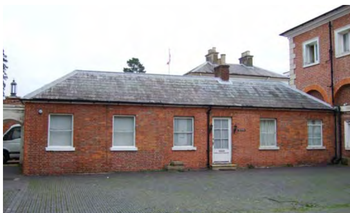
Plate 14 The same wall as shown in Plate 13 showing the appearance as in 2007
