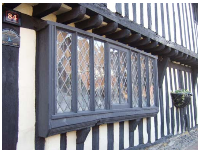
Plate 2 Oriel window serving hall
