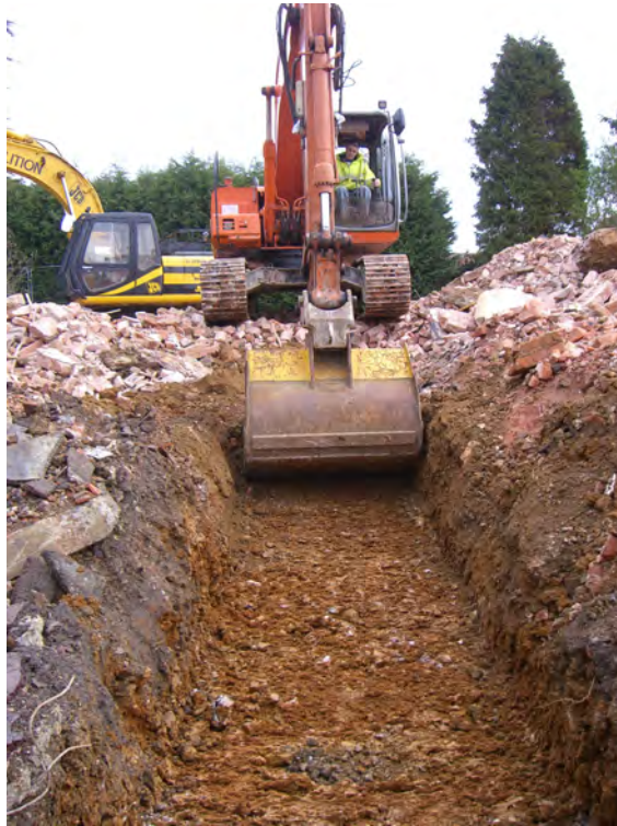
Fig. 3: Working shot of excavation of trench 2
