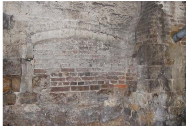
Plate 12 Arch carrying wall over site of former oven
