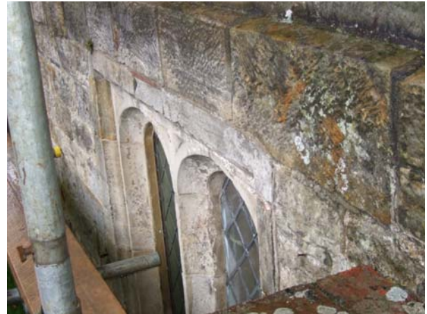
Plate 4 Window at basement level
