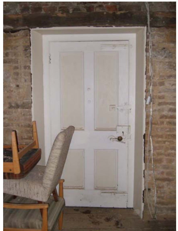
Plate 3 Interior of front door
