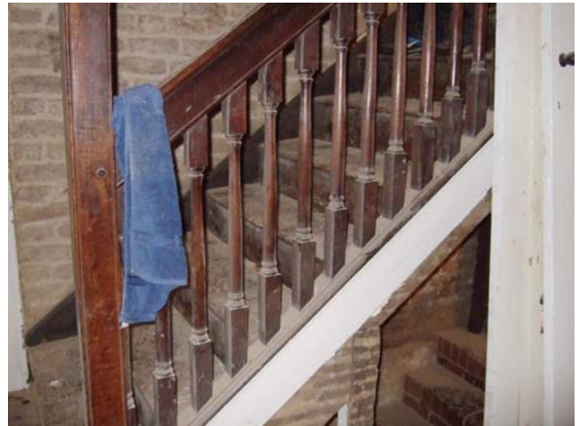
Plate 11 Balustrade to main staircase
