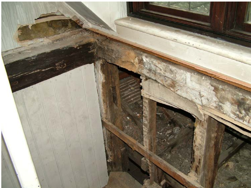
Plate 2 Attic stairs showing tiebeam jointed to wallplate in level assembly.
