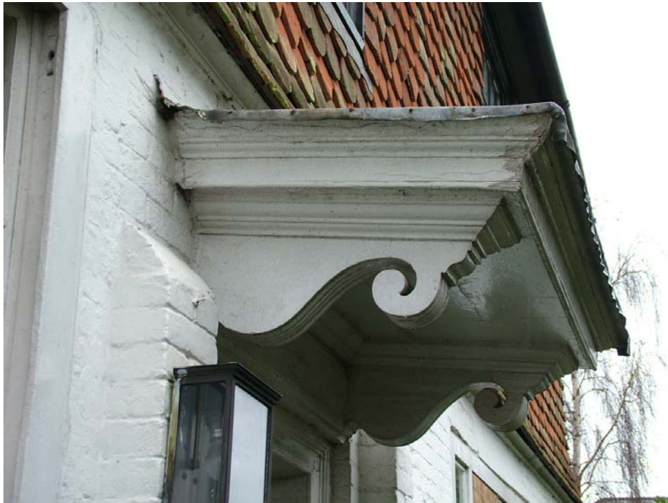
Plate 9 Detail of hood over entrance doorway.
