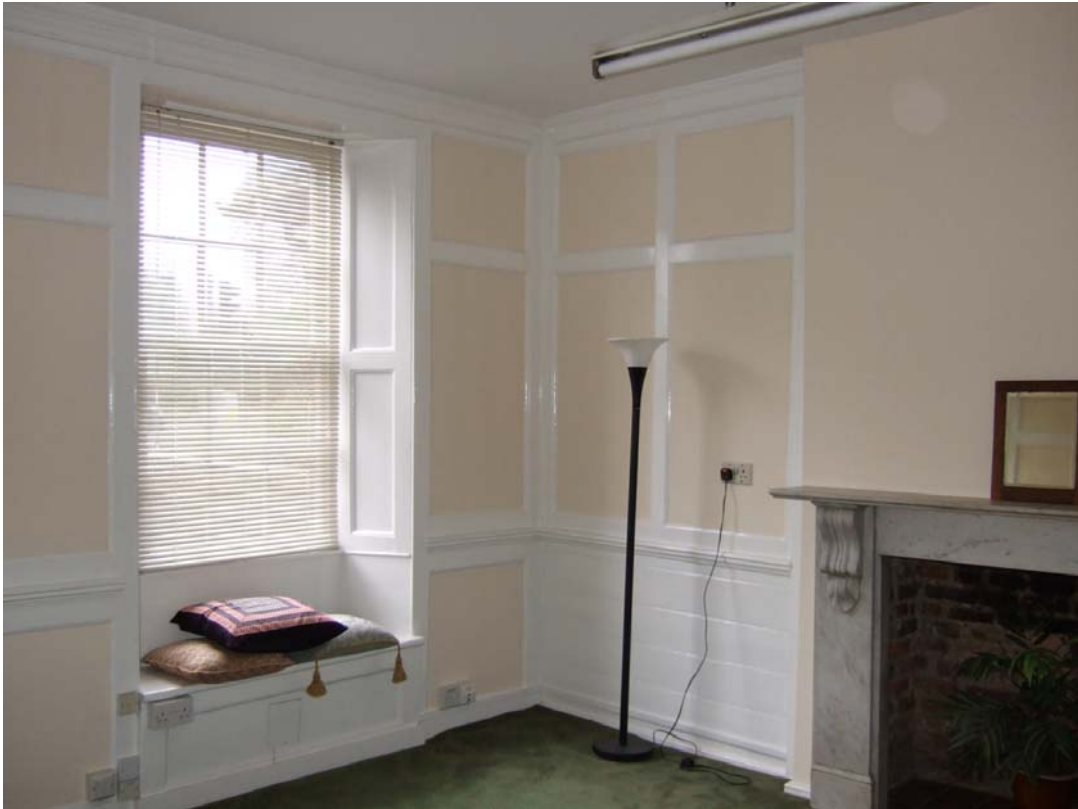
Plate 3 - Panelling, window seat and shutters in ParLOUR.
