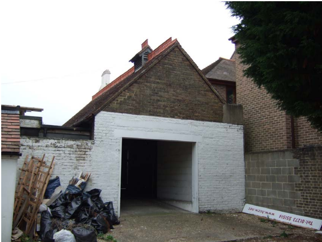
Plate 13 - Coach house viewed from north showing intruded entrance.
