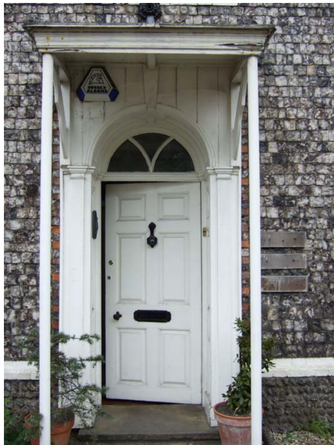
Plate 2 - Detail of front door.
