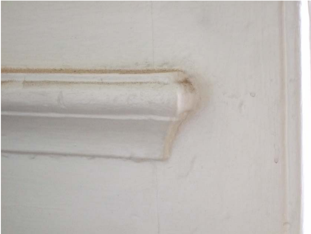
Plate 7 - Dado rail within Parlour Chamber.
