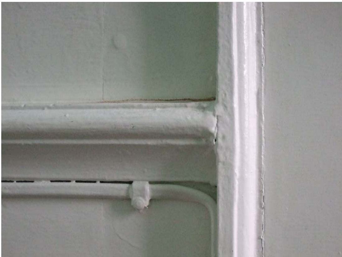
Plate 8 - Dado rail and architrave to closet doorway within Parlour Chamber.
