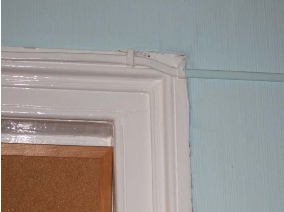
Plate 9 - Door frame and architrave to closet doorway.
