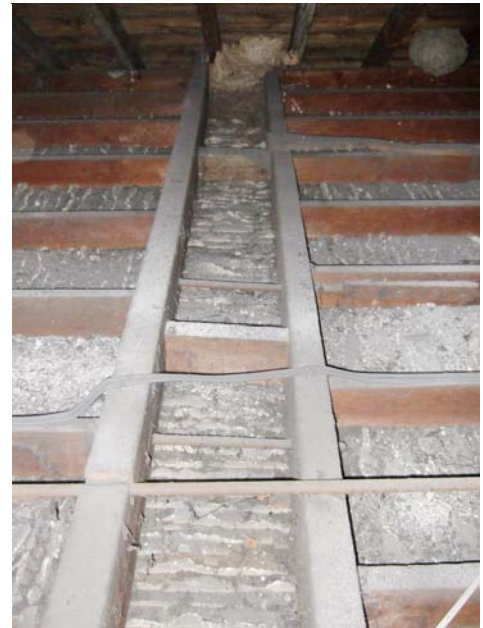
Plate 9 'Composite tiebeam' in roof
