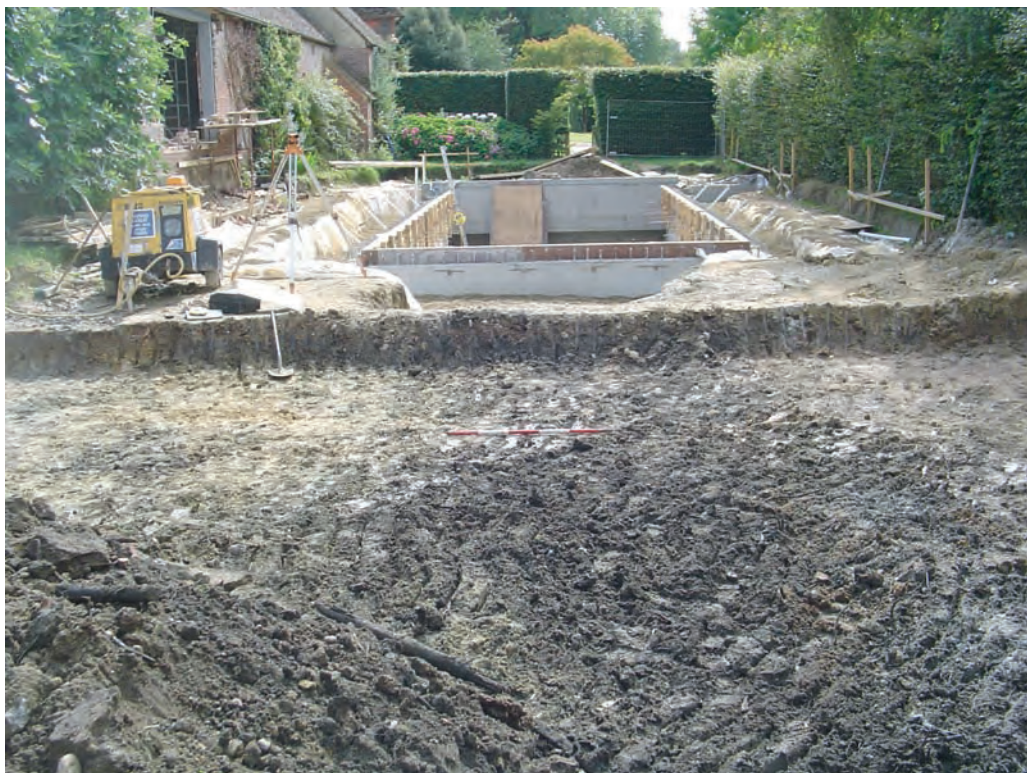
Plate 2: Area of Glass House
