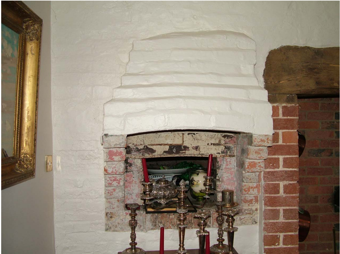
Plate 4 Replacement bread oven within Bakehouse.
