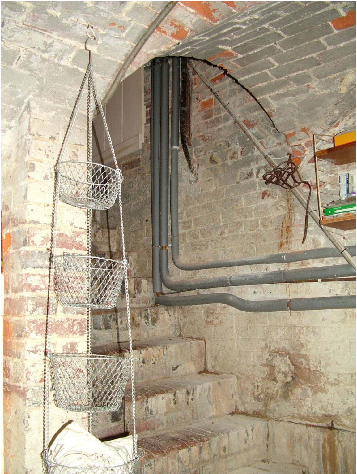
Plate 2 Brick arch at base of steps leading into cellar.
